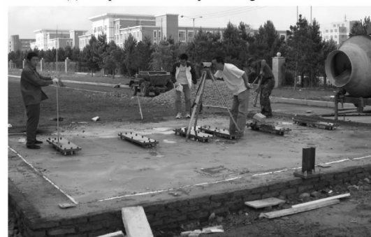
(b) Measure planes error of pre-embedded piece
