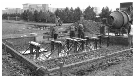
(a) Fix pre-embedded piece of ground base
